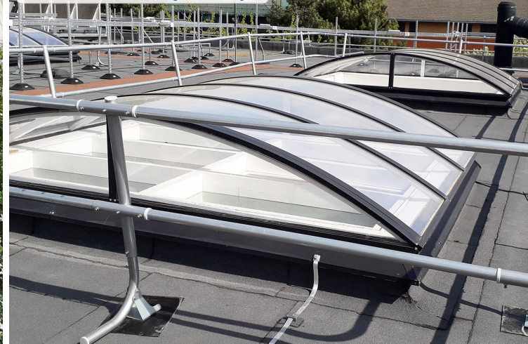
Moj: Leicester Court double-glazed roof lights
