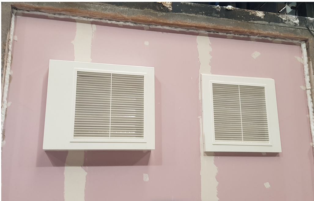
Fire Integrity Test installation of ATG-FSS at Element WarringtonFire
